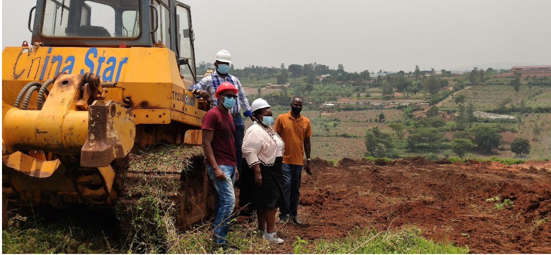
First construction work for the new stove factory
