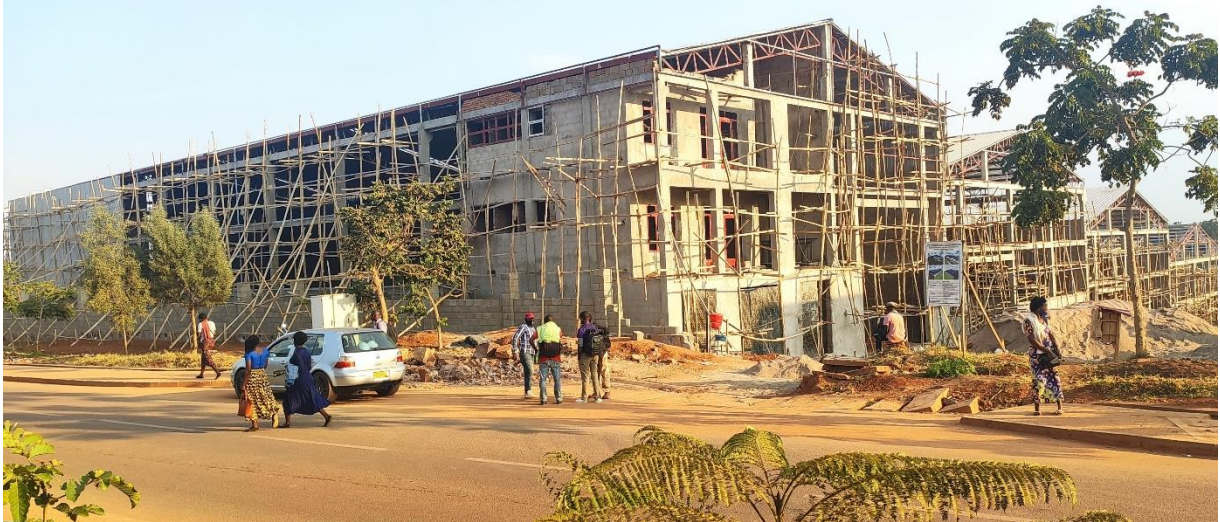
New Factory Building in Kigali
