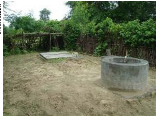
Fig: Biogas Digester in Operation
