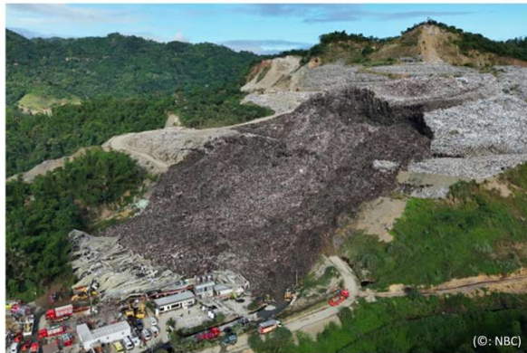
Landfill Slide at Binaliw Landfill, Cebu, 08/01/2026
