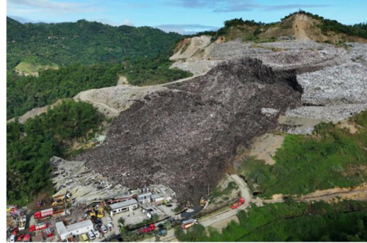
Landfill Slide at Binaliw Landfill, 08/01/2026
