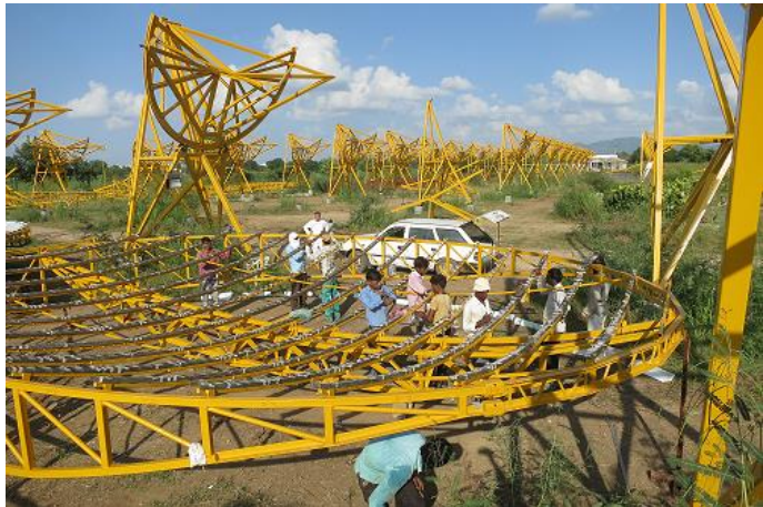
Figure 5: Setup of one of the steel frames for the mirrors.
