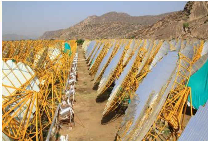
Figure 6: Side view on the solar dishes and cavity receiver.
