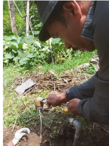
Defective gas pipes are replaced
