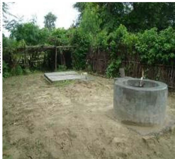
Fig: Biogas Digester in Operation
