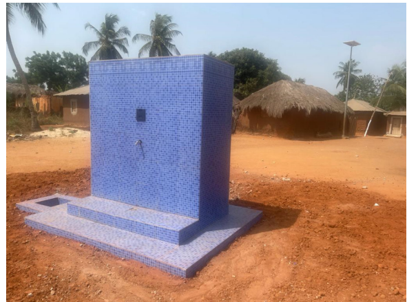
A water kiosk in Adjegan
