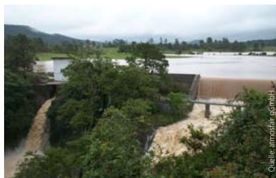
Honduras: Small hydroelectric plant
