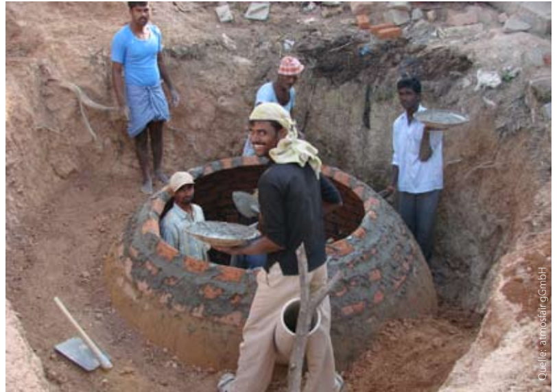
Cow dung is fermented in underground biogas digesters, producing an almost odorless gas.
