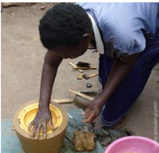
Building a wood-fired clay oven in Malawi
