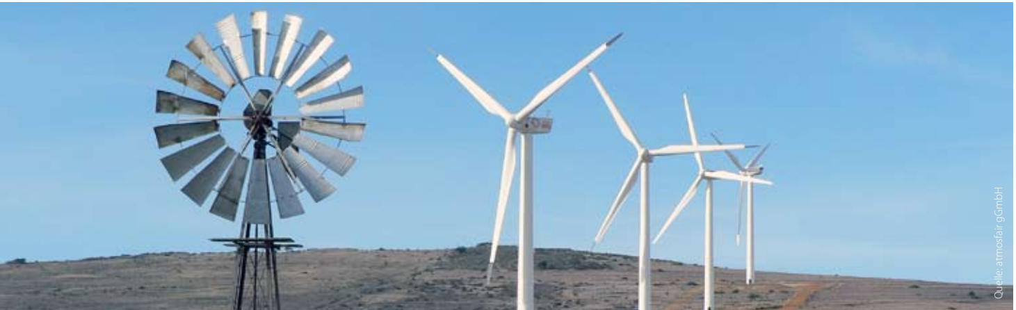
The Darling Wind Farm has been generating climate-friendly electricity since 2008
