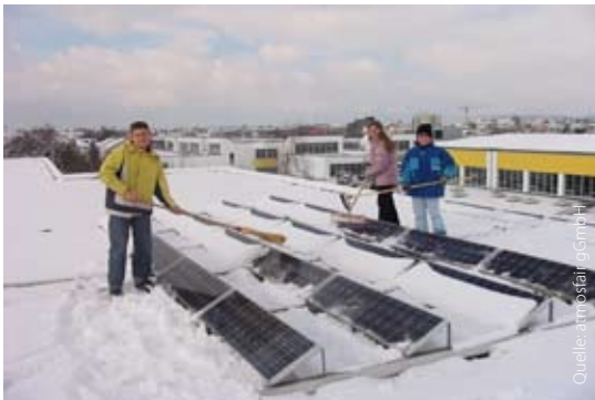
The solar panels produce green electricity in winter as well
