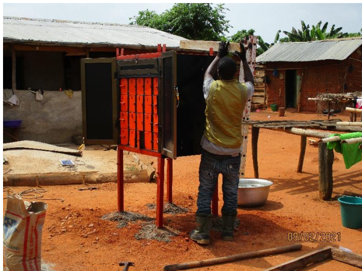
Construction of a solar kiosk
