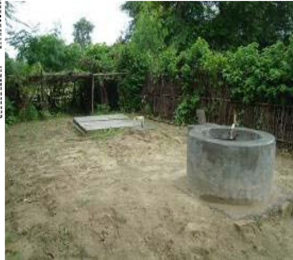
Fig: Biogas Digester in Operation
