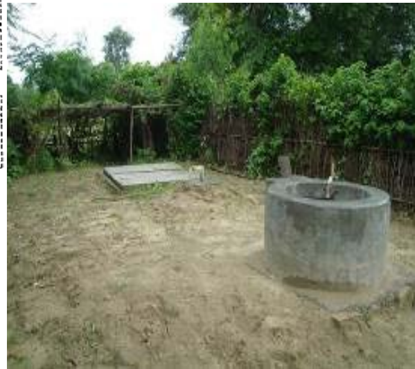
Fig: Biogas Digester in Operation
