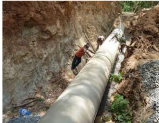
Workers in Sri Lanka laying water line pipes.
