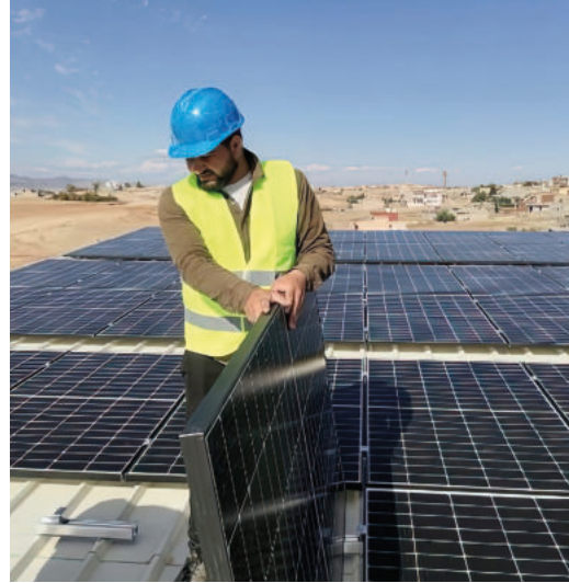
Basem, an electrician from our partner TopWay, installs a solar module on the school roof
