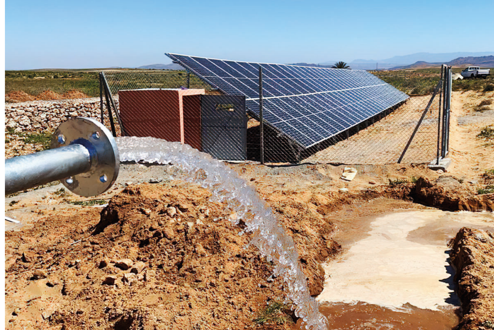
The water pumps are operated entirely with solar energy.
