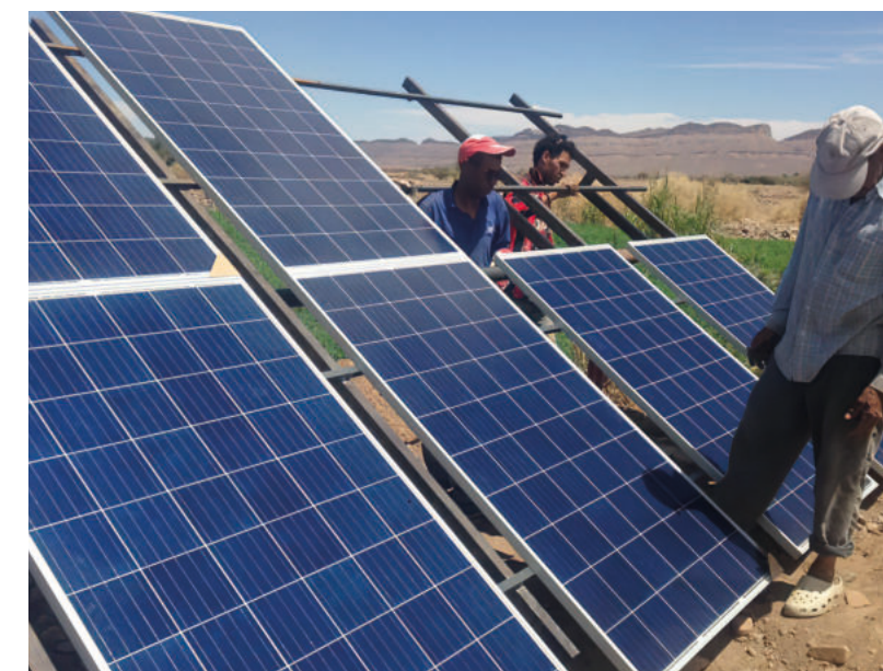
Local installers assembling a 9.8 kW solar installation.
