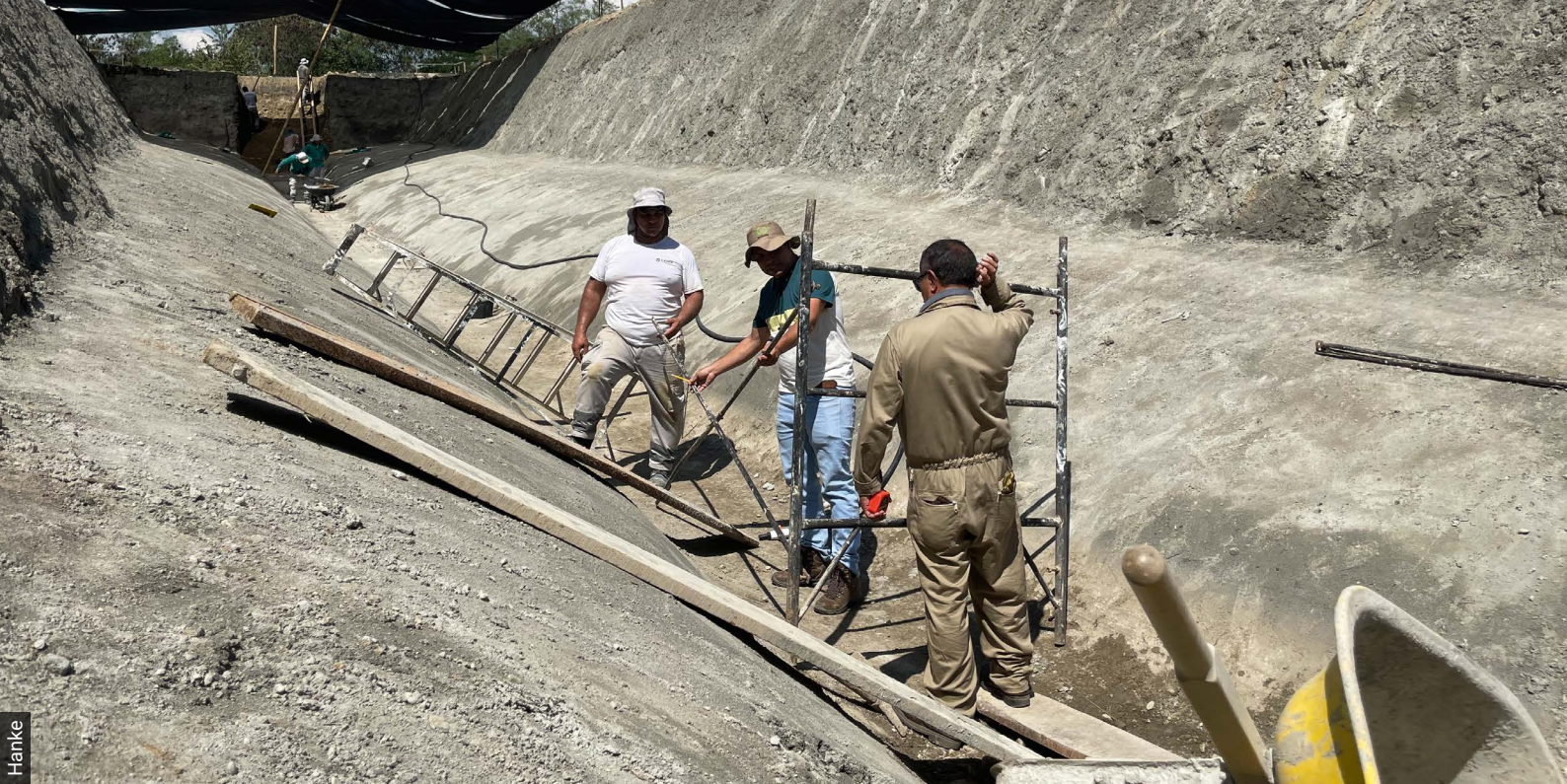
Construction workers are lining the biogas plant pit with concrete.
