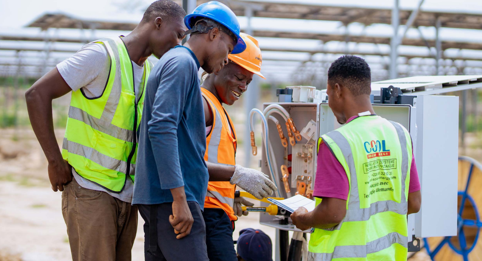
■ SUNtec technicians prepare Dalavé's agri-photovoltaic system's connection to the Togolese power grid.
