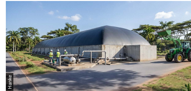
From right to left: Tobias Hanke, John Castillo (SENA) and the staff at Hanke are building a biogas plant that is the first of its kind in Colombia (see illustration). The membrane roof seals the pit airtight, allowing the biogas produced to be captured and used in a controlled way.
