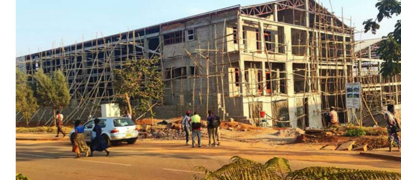
Progress on construction of the new building in Kigali, Rwanda @atmosfair
