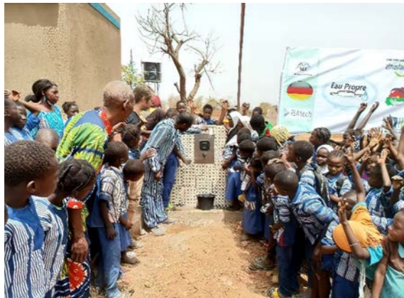
Inauguration of the first solar-powered water treatment plant with distribution network in Dedougou @atmosfair
