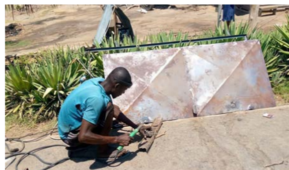
Here we see an ANKA employee installing the distribution grid ©ANKA metal worker Tovonance at work ©ANKA
