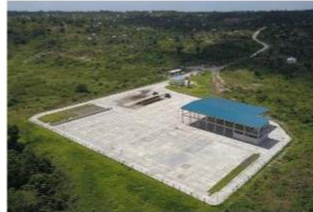
Compost Plant, Dar es Salaam
